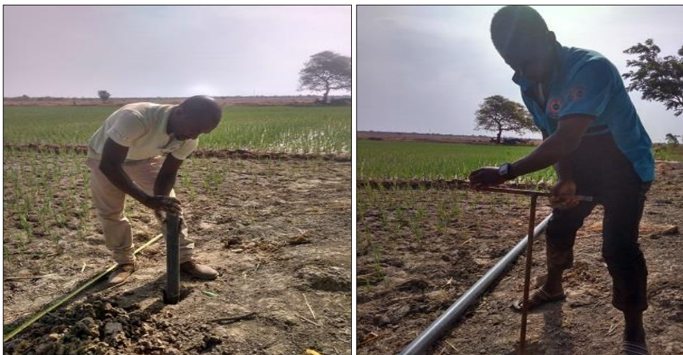
Plate 3.3: Installation of Observation Wells in the Irrigable Area
