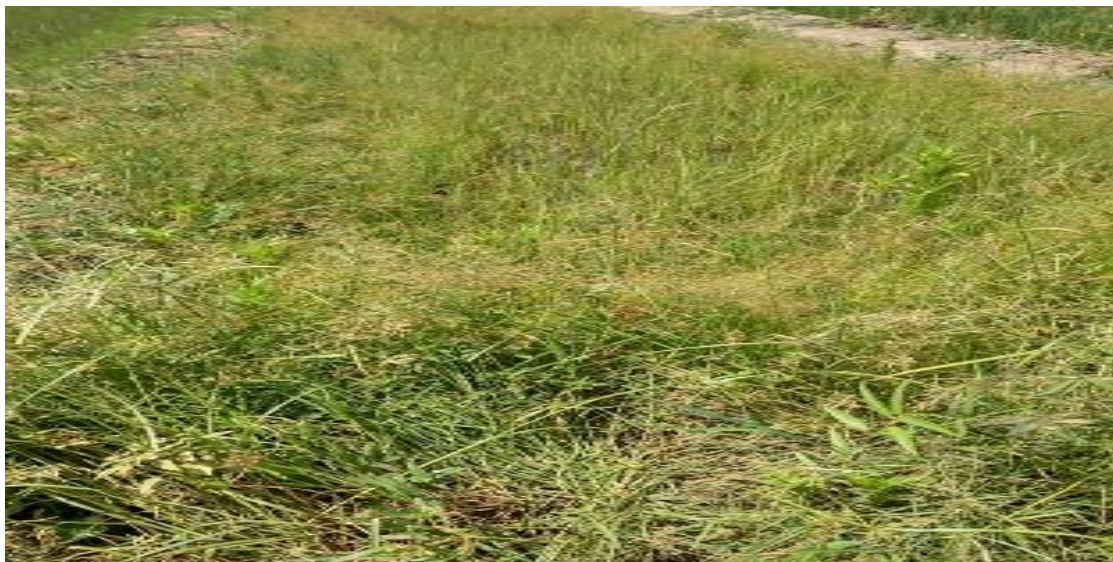
Plate 4.2: Condition of Lateral/Collector Drains of Bontanga Irrigation Scheme
